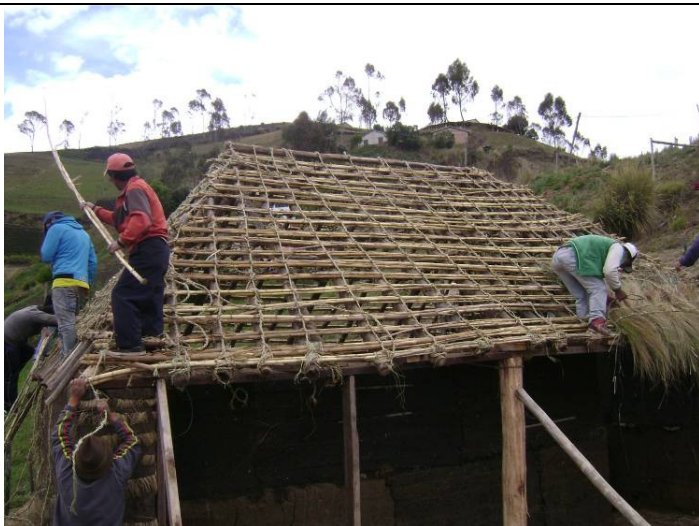
Esperanza, August 2013. Construction of a traditional 'choza', and adobe-walled, thatched-roof dwelling.
